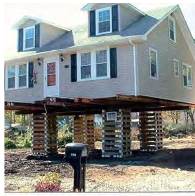
House on temporary bearers
